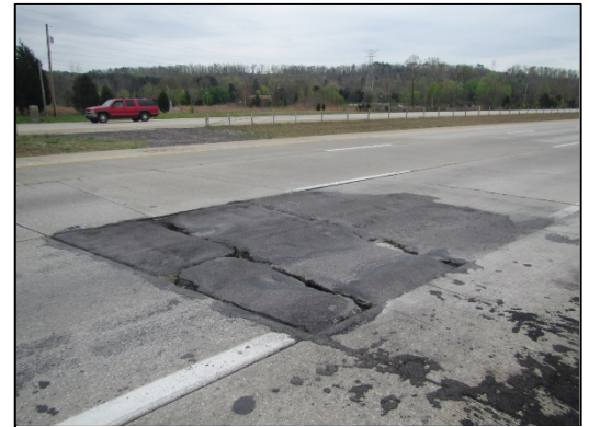
Example I-65 Pavement Repair
